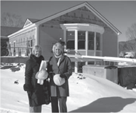
Board member Barbara O'Connell (left) and Program Committee member Ann Shriver Sargent admire the progress made on the construction of the Education Center.
