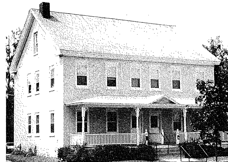
(figure 1) Birthplace of Grace Goodhue at 315-317 St. Paul Street, Burlington, Vermont
